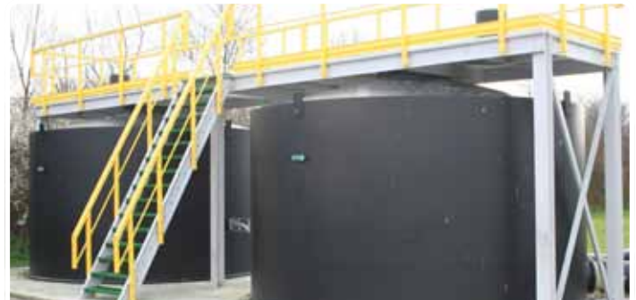
Entrance platforms Water treatment plant
