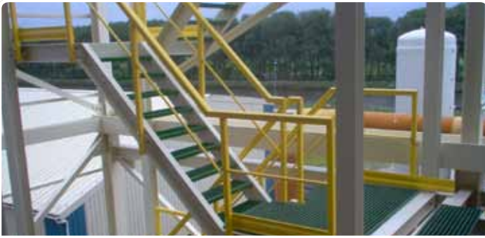
Customized secondary structures Fertilizer plant
